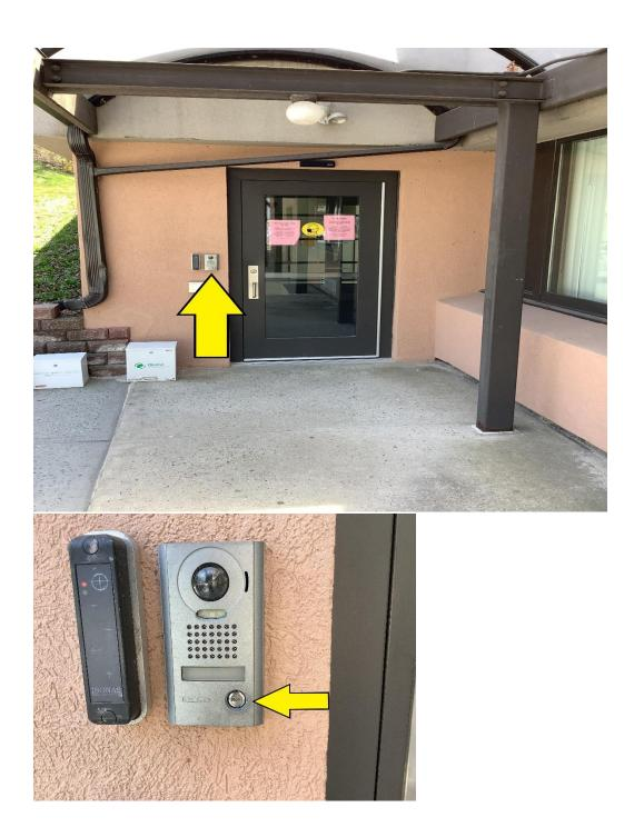
When we approach the door, we push a special button which will unlock the door.
